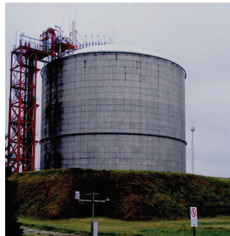
Fig. 1. Atmospheric 30.000 m 3 LPG tank
